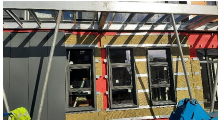
Three simple shrouds manufactured for the demonstrator building
